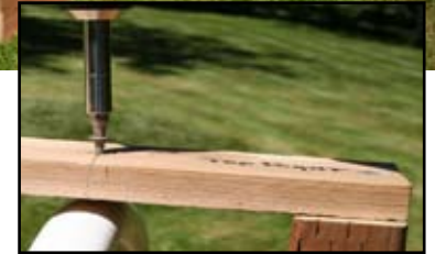
Figure 5 insert. Secure the backbone to the C board and the rib.
