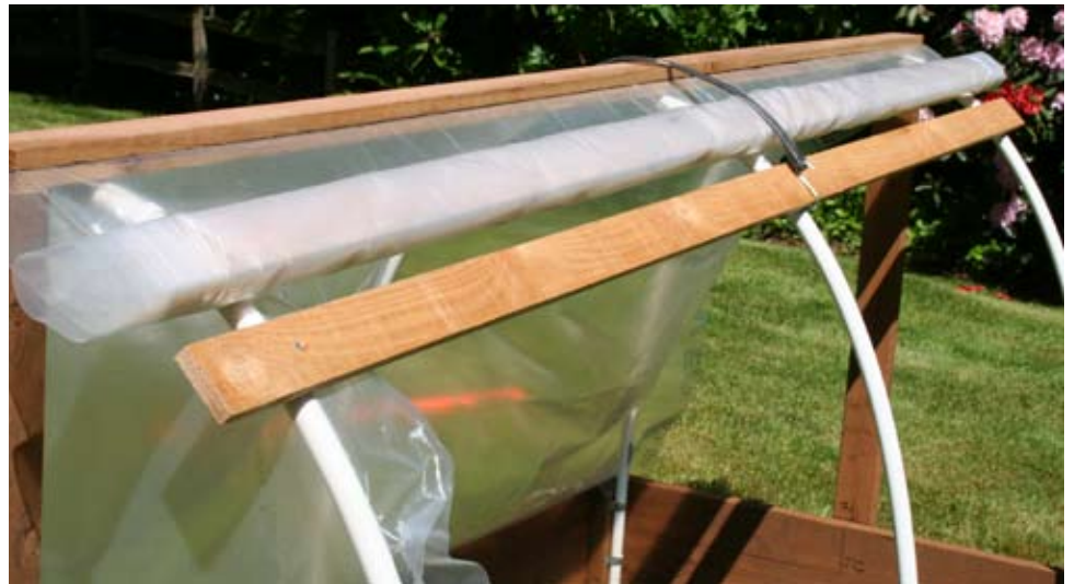
Figure 11. A D board attached to all the hoops 10 inches below the backbone on each side gives the structure extra strength and support.
